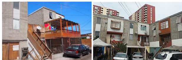
Permanent (left) and temporary (right) frontal extensions in courtyards.
