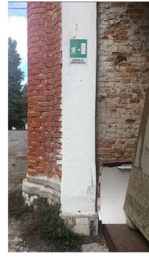
B. The joint between the S.Donato Cathedral column and wall of barrack before 1786, can be seen here. (Exterior View)
