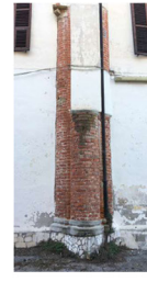
C. The joint between the S.Donato Cathedral column and wall of barrack before 1786, can be seen here. (Exterior View)
