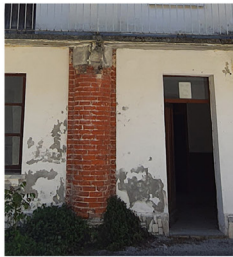
A. Cathedral column noticeable on facade of other side. The walls added in order to make biletts belong to period before 1786.
