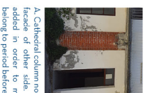
B. The joint between the S. Donato Cathedral column and wall of barrack before 1785, can be seen here. (Exterior View)
