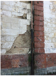
E. View of the Galliano Barrack where it is evident that the material used is different as compared to other walls (from other phases).
