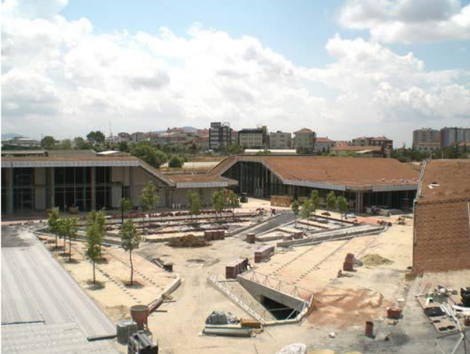
Fig. 54 layering of substrate during construction of green roof Retrieved from (ZinCo, 2022)
