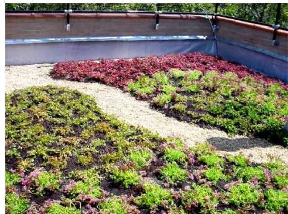
Fig. 4 Extensive Green roof on 18 th street residential building in New York, USA Retrieved from greenroofs.com Oct. 2021
