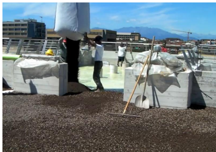
Fig. 39 Installation of substrate layer on rooftop of 25 Verde. Retrieved from Lineeverdi.com (2022)
