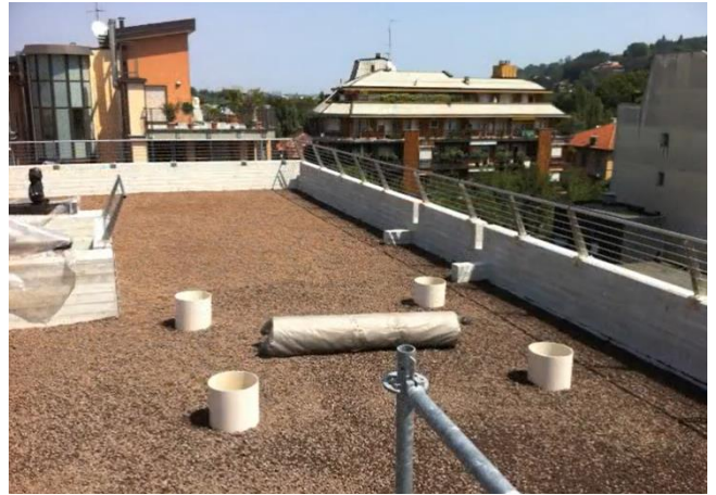
Fig. 41 Installation of substrate layer on rooftop of 25 Verde. Retrieved from Lineeverdi.com (2022)
