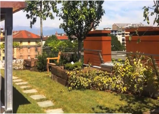
Fig. 42 Intensive green roof installed on rooftop of 25 Verde with seating area. Retrieved from Lineeverdi.com (2022)
