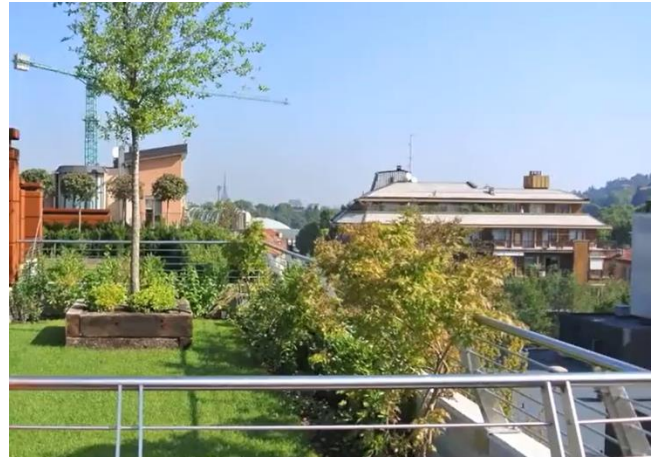
Fig. 43 Fig. 42 Intensive green roof installed on rooftop of 25 Verde. Retrieved from Lineeverdi.com (2022)
