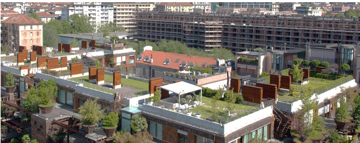
Fig. 35 Green roof of 25 Verde. Retrieved from (due.to.it, 2022)
