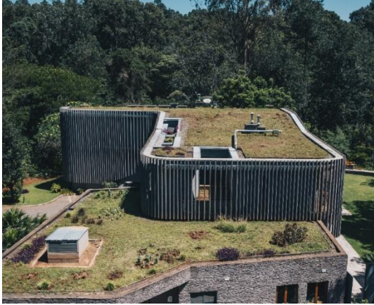
Fig. 24 French embassy residence green roof (Monocle, 2021)
