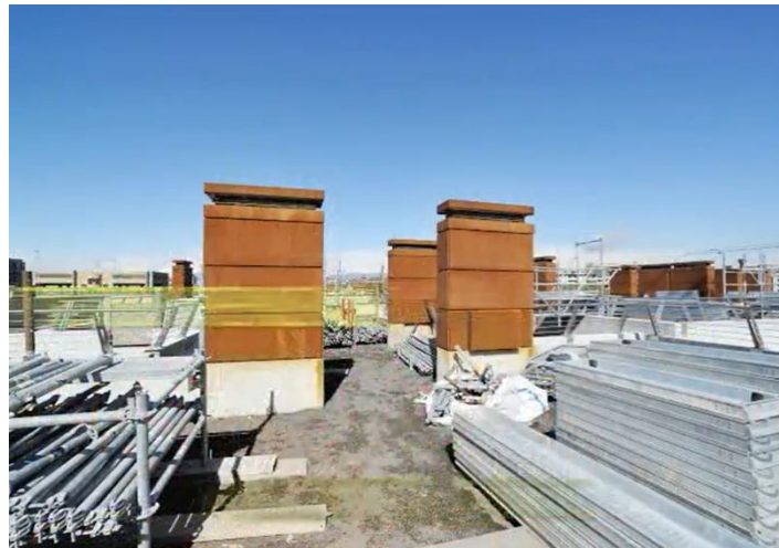
Fig. 38 25 Verde roof before construction of green roof. Retrieved from Lineeverdi.com (2022)
