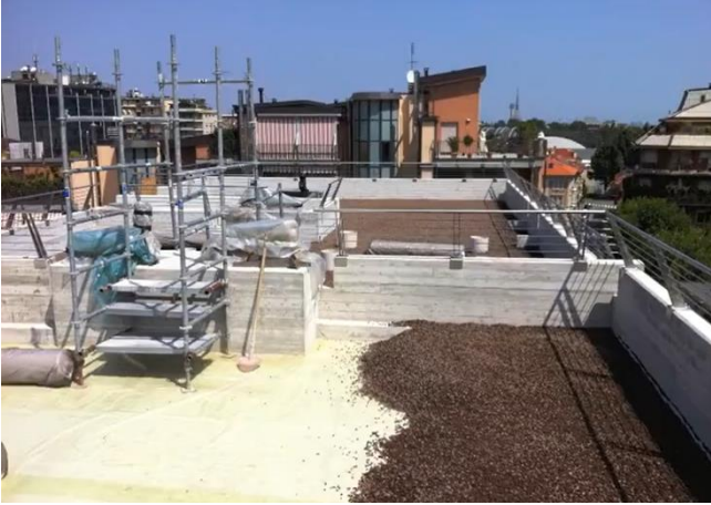
Fig. 40 Installation of substrate layer on rooftop of 25 Verde. Retrieved from Lineeverdi.com (2022)
