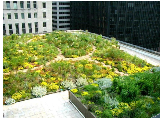
Fig. 5 Semi-intensive Green roof on Chicago City hall, Chicago, USA Retrieved from greenroofs.com Oct. 2021
