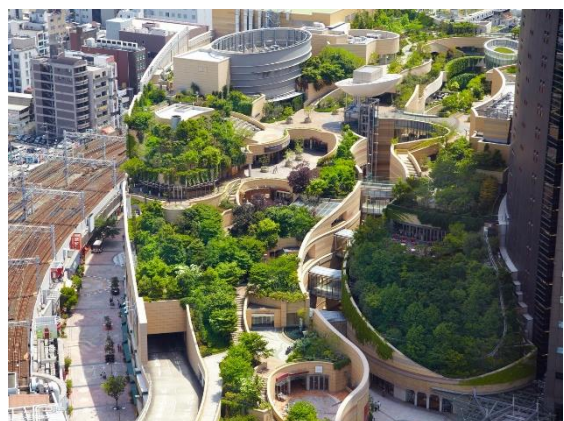
Fig. 6 Intensive Green roof, Namba Parks, a retail and office complex in Osaka, Japan Photo by Yuji Kotani, retrieved from guardian.com, Oct. 2021
