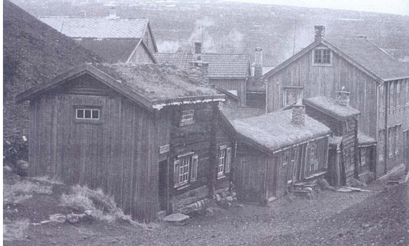
Fig. 1 Miners' houses with turf roofs dating from the 17th to the 19th century in Røros, in Sør-Trøndelag, Scandinavia (Donnelly, 1992)
