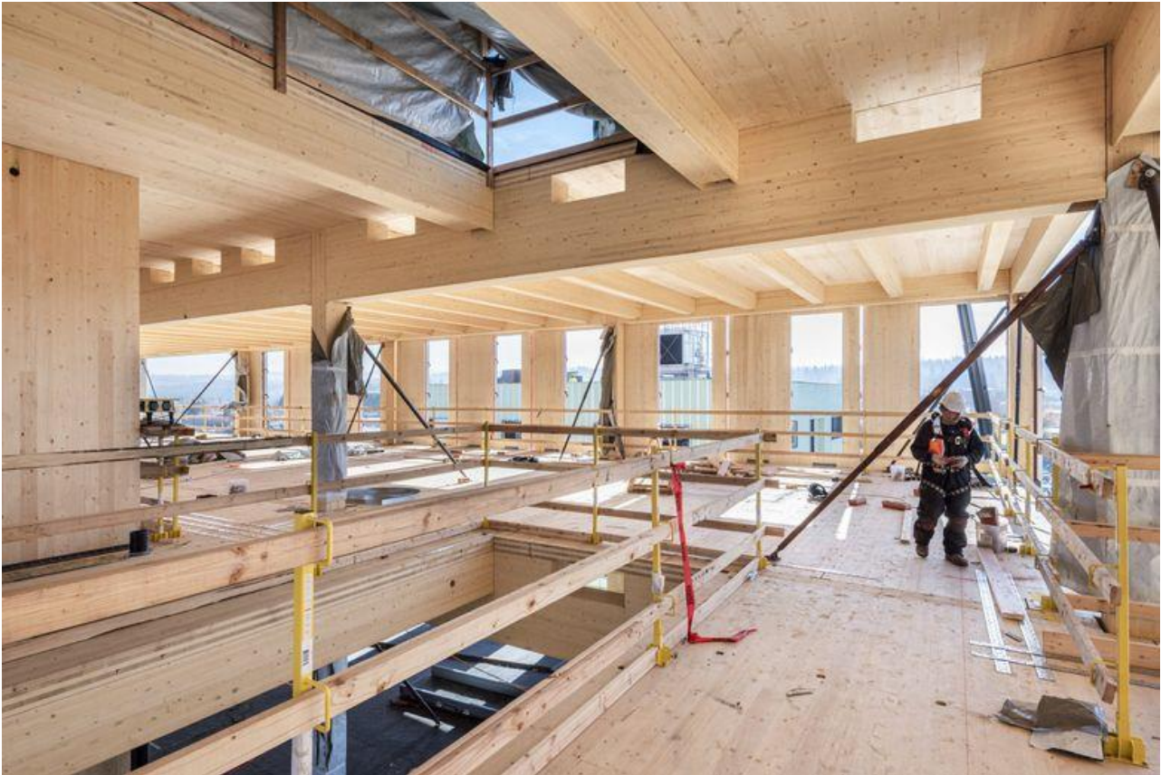
Figure 7. Katerra construction site (Seattle Times business, 2021)
