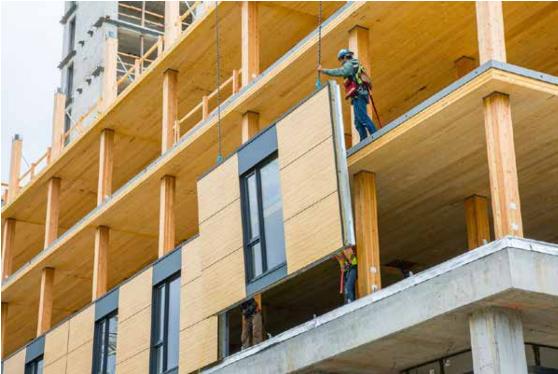
fig 1.2.6 - Assembly of prefab wall panels on site Source - Think Wood - Brock Commons Tallwood House
