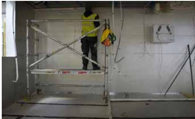
fig 5.2.22 Interior panelling and cables put in place
