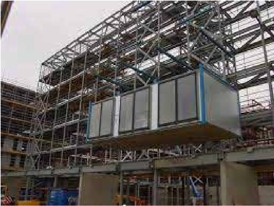
fig 3.8.6 Installation of modules behind external steel framework at MoHo Manchester Source - ED014, Light steel framing and modular construction series by R M Lawson
