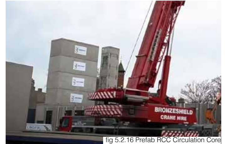
fig 5.2.16 Prefab RCC Circulation Core
