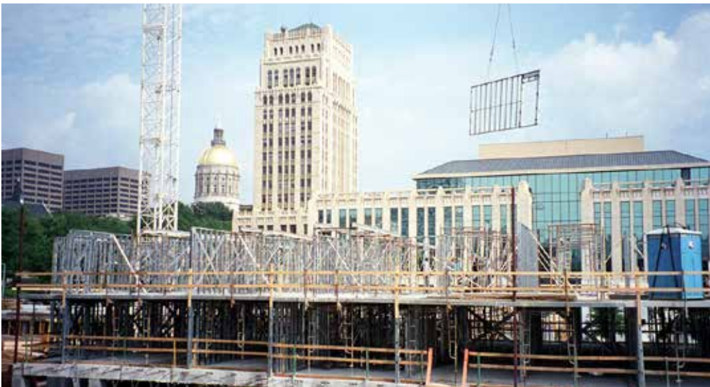
fig 4.1.2 On Site construction and Assembly of Prefab Steel Components
