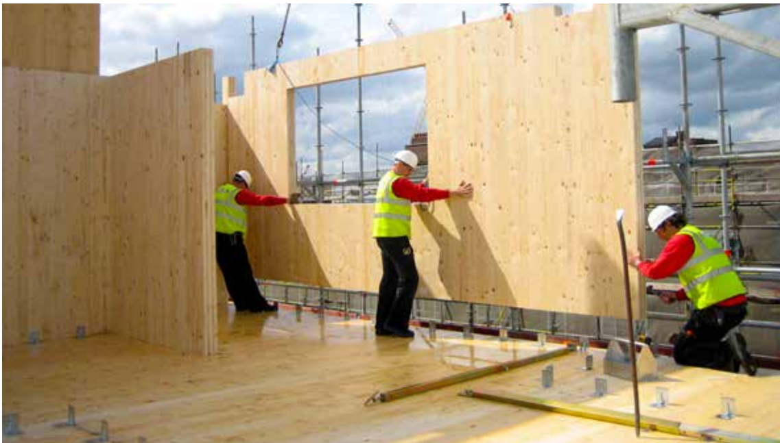
fig 3.1.5 - CLT Panel Assembly On-Site Source - Simpson Strong Tie
