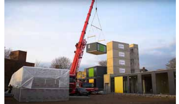
fig 5.2.29 Modules assembled to location with crane
