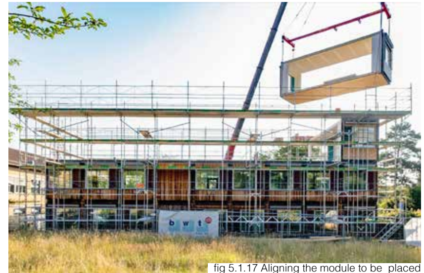
fig 5.1.17 Aligning the module to be placed
