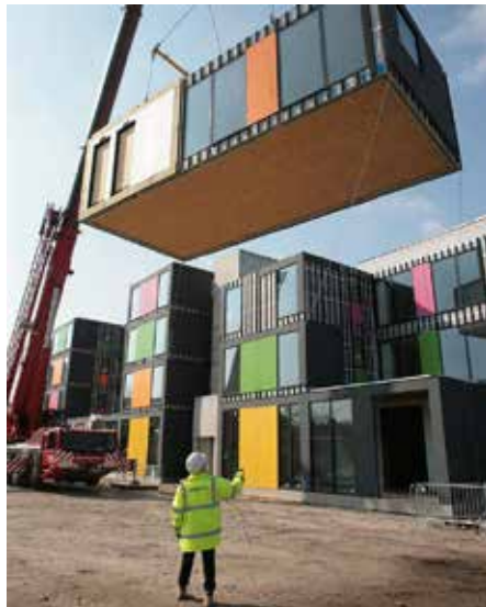
fig 5.2.13 Lifting the module to place on precise location
