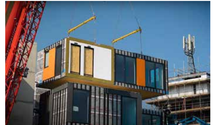
fig 5.2.32 Assembled blocks ready for facade treatment
