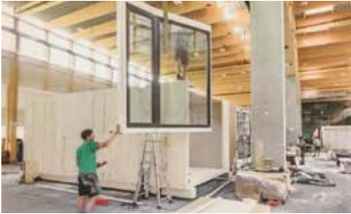
fig 3.5.7 Window mounting.
