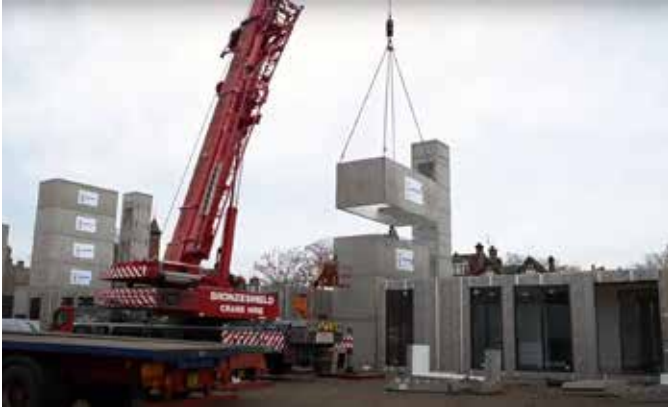
fig 5.2.27 Precast Concrete blocks stacked for stairwells
