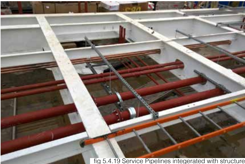
fig 5.4.19 Service Pipelines integrated with structure.
