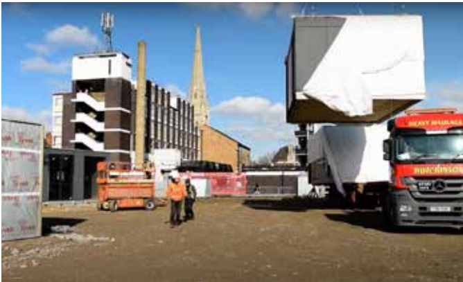
fig 5.2.30 New modules ready on site to be assembled
