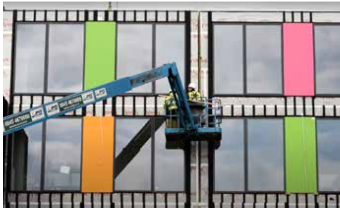
fig 5.2.31 Exterior facade cladding and sealing junctions
