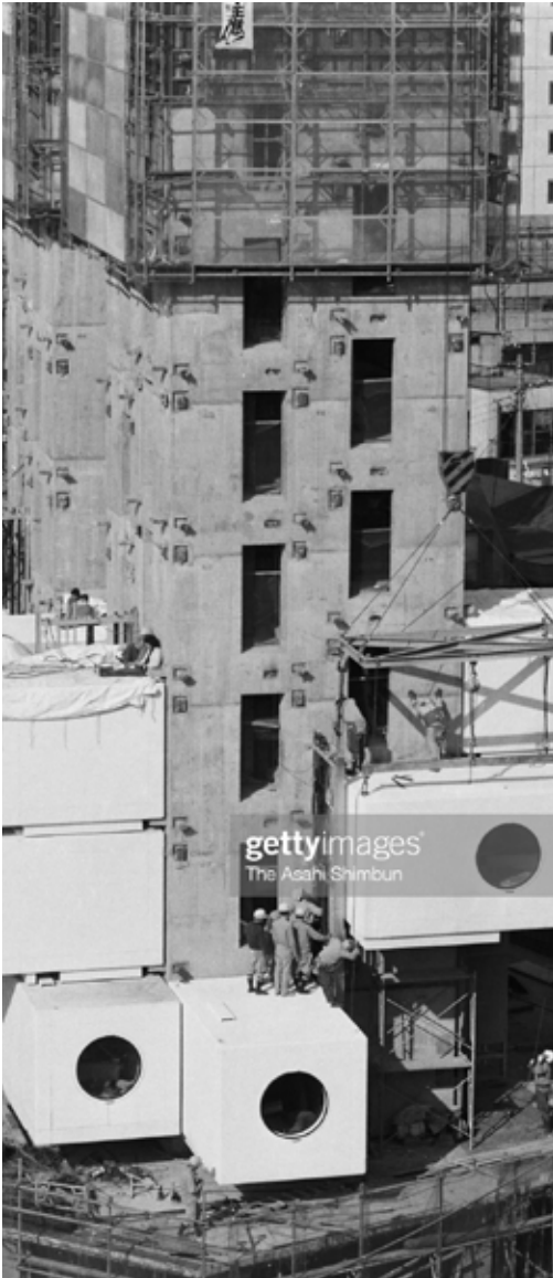
fig 1.1.1 Nakagin Tower - On site construction process Source - Getty Images
