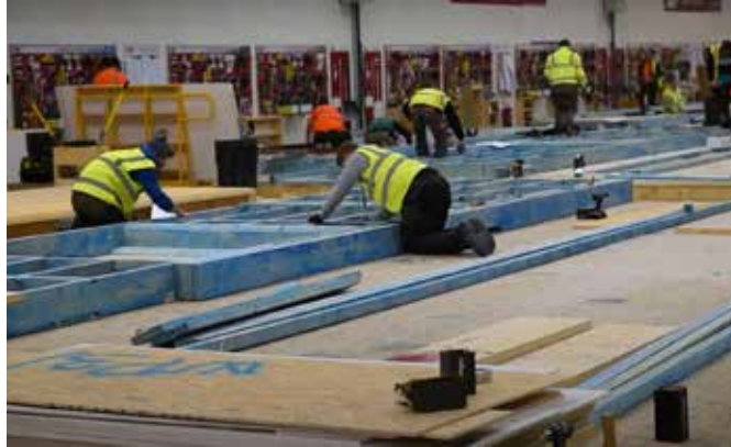
fig 5.2.19 Preparing the timber frames for walls
