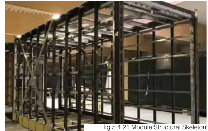
fig 5.4.21 Module Structural Skeleton
