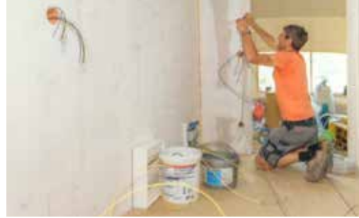
fig 3.5.6 Electrical piping and insulation.
