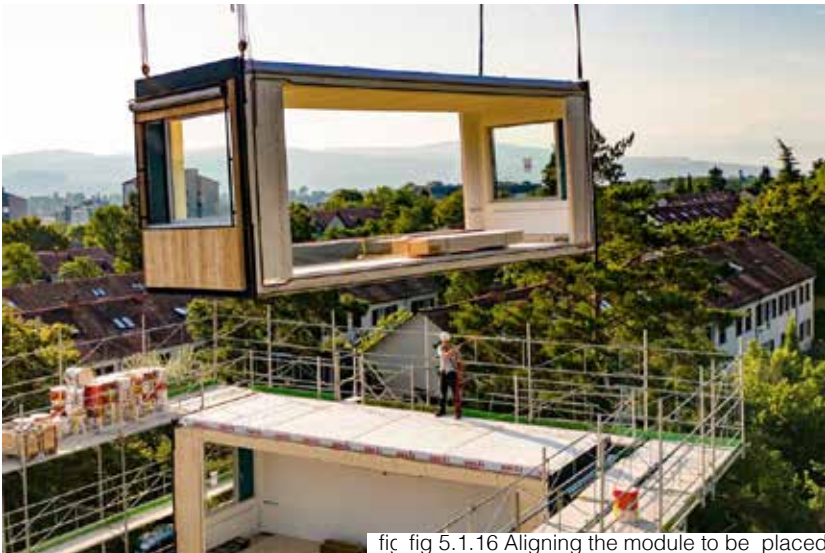
fig 5.1.16 Aligning the module to be placed
