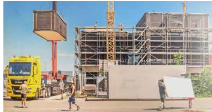
fig 3.5.15 Hotel Nordlingen 2018 .Mounting of room modules.
