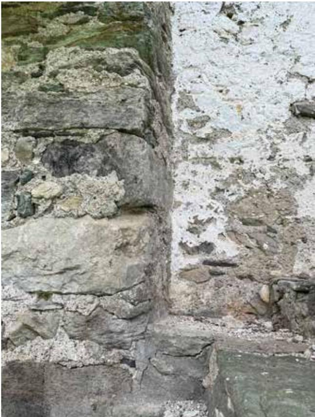
In the third phase we can identify a difference in the type of stone used between the wall in the left and the one in the right. This makes us understand that it was a volume in addition to the original body, also because it is pushed back by a couple of centimeters. This was most probably due to the expansion of the family.
