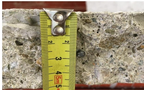
Figure 9: Depth of Reinforcement
