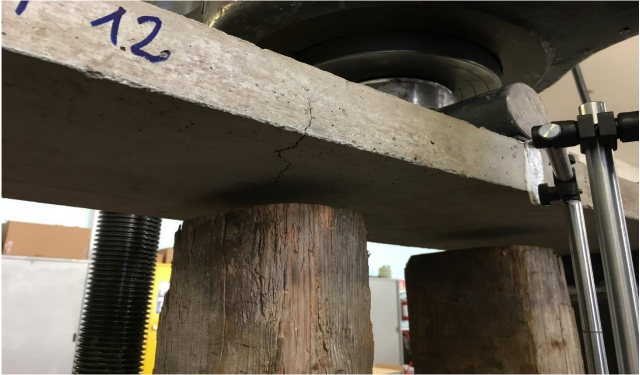
Figure 20: Visible Crack on RFRC
