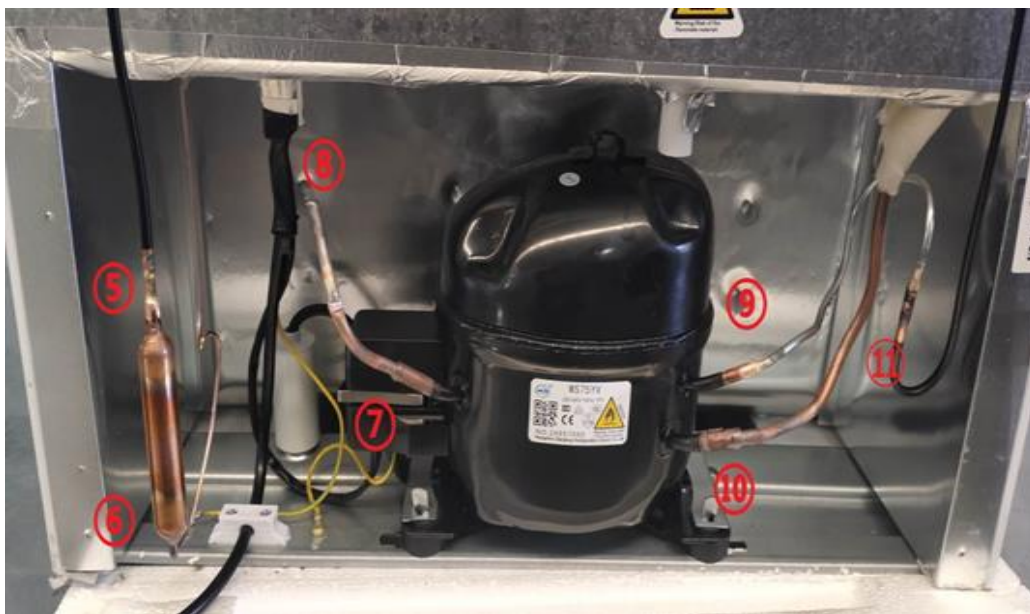
Fig 18. Welding points BI Combi Static II
