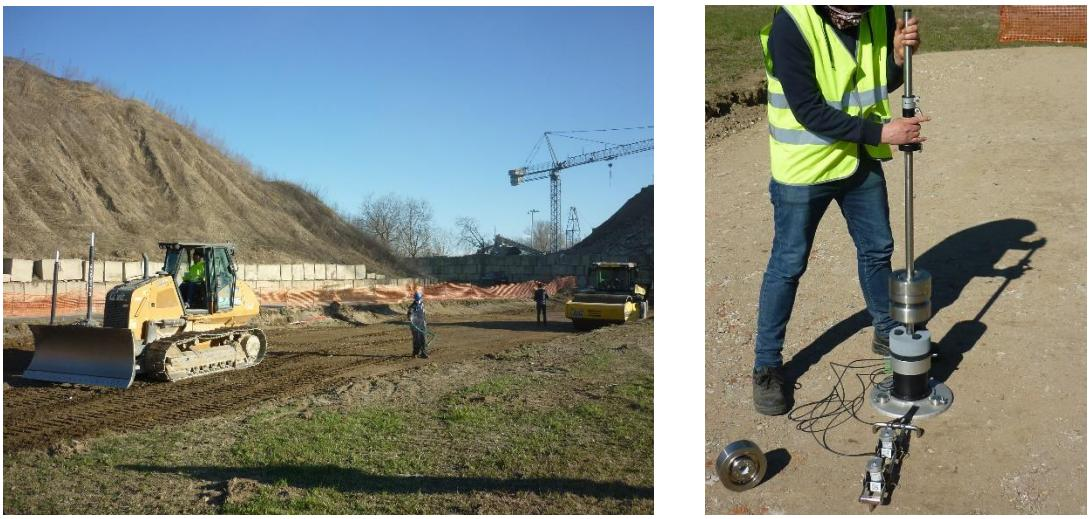
*Figure 26: Placement of layer 1 (a); Test execution on layer 1(b).*
