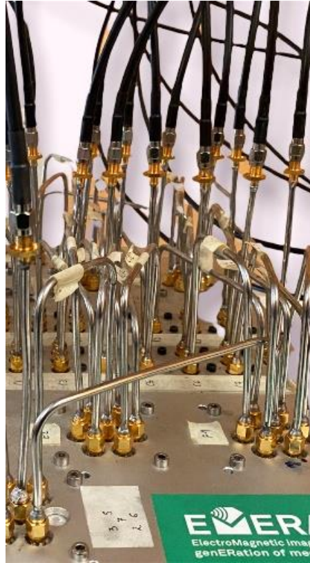
Figure 3.20. Semi-rigid coaxial cables connected to the switching matrix and flexible coaxial cables connected to the antennas.
