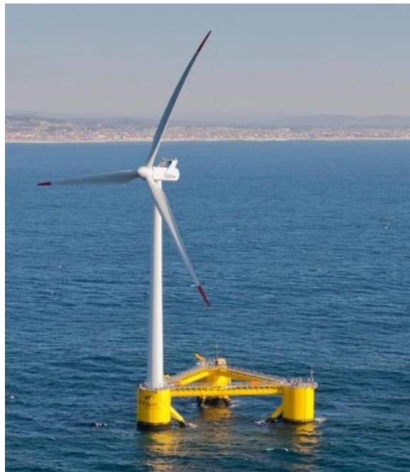
Figure 2.6 Semi-submersible substructure concept
