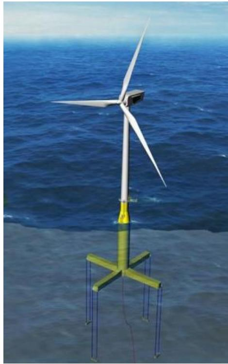
*Figure 2.7 TLP structure design*
