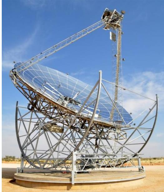
Figura 29 Parabolic Dish Collector[64]
