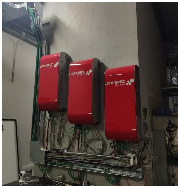
Figure 4-8 Installed inverters
