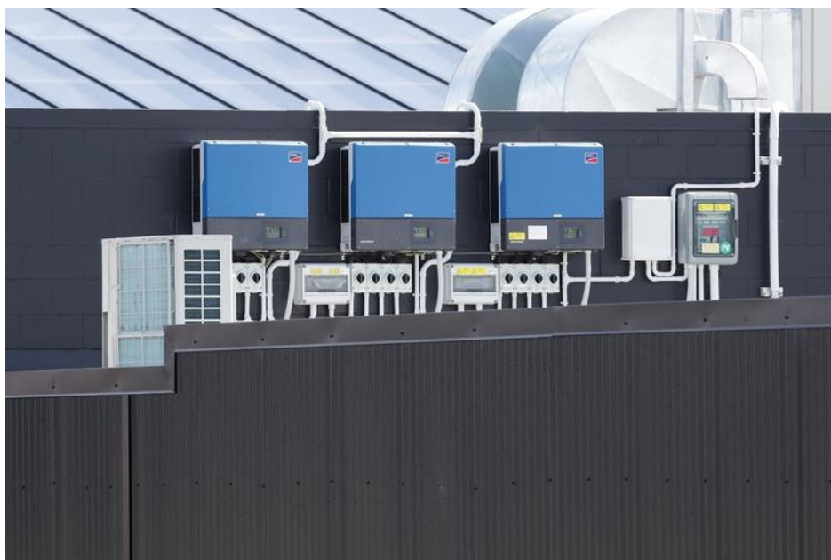
Figure 3-10 Inverters and smart meters used [84]
