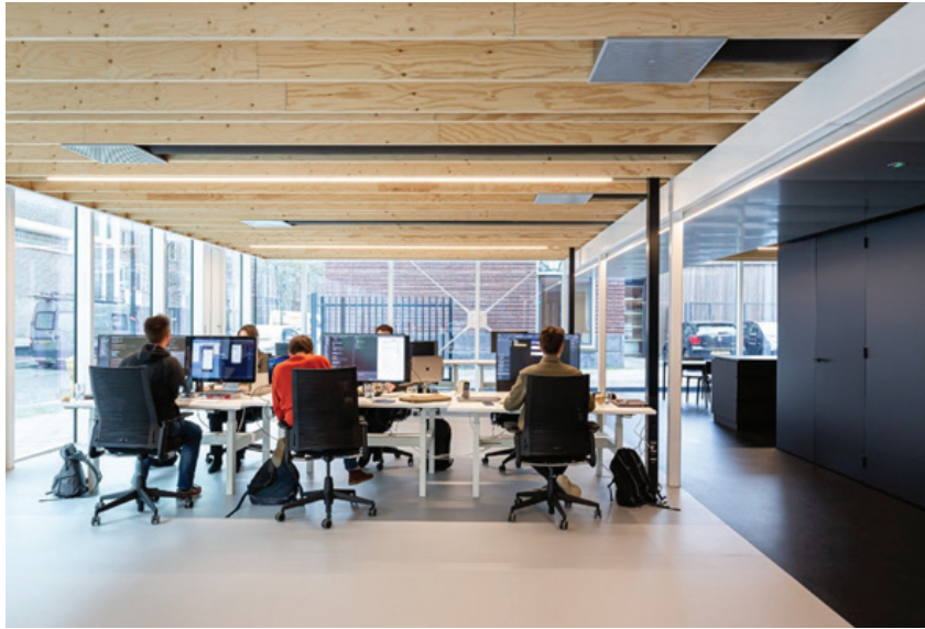
Image 10. Part of aesthetics of the building is its simple prefabricated LVL floor structure (cepezed.nl).
