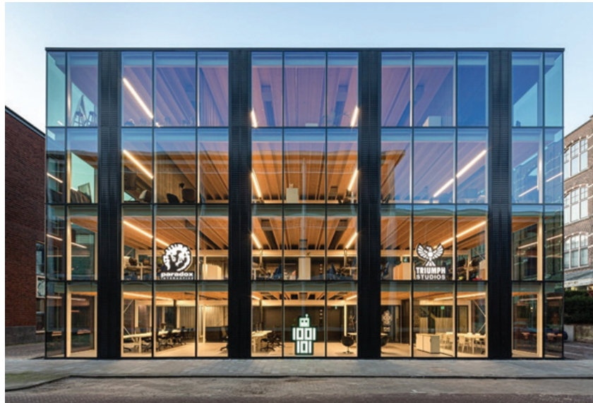
Image 08. Building D's façade is mostly transparent and its frameless structure reduces the material use (cepezed.nl).
