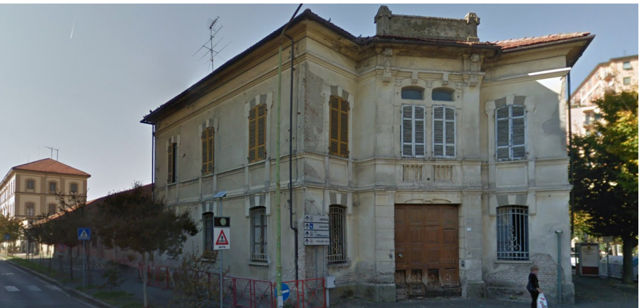
vista ingresso principale deposito https://www.google.com/maps/@44.7626162,8.7949391,3a,75y,263.59h,92.34/
