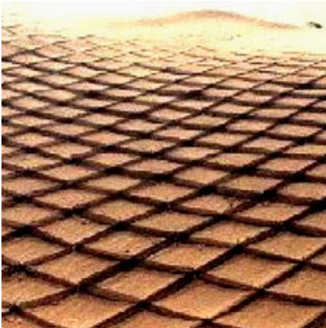
Fig.1 Semi-buried sand barriers in a checkerboard pattern. In Jianjun Qu, et al. (2007) Field observations on the protective effect of semi-buried checkerboard sand barriers, Geomorphology , 88:194
