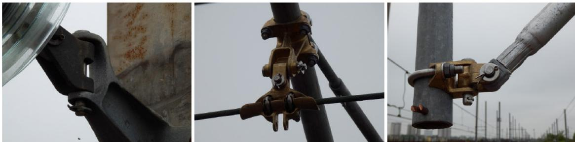
*Figure 1. 5 Joints between bracket and mast (left side), messenger wire and bracket (centre) and registration arm and steady arm (right side). From (Vo Van, 2016).*
