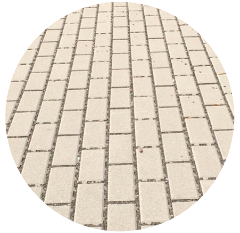
Permeable pavers in rectangular tiles Available in: https://www.epa.gov/soakup-therain/soak-rain-permeable-pavement
