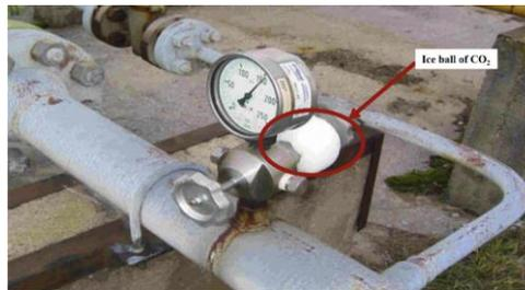
Figure 8. Formation of solid CO<sub>2</sub>/ice around a pressure gauge during leakage of CO<sub>2</sub> [5].
