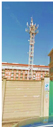
Figure 3-21, example of 3 sides lattice tower
