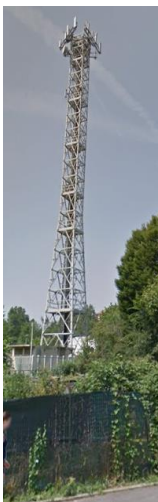
Figure 3-19, example of Pyramid lattice tower
