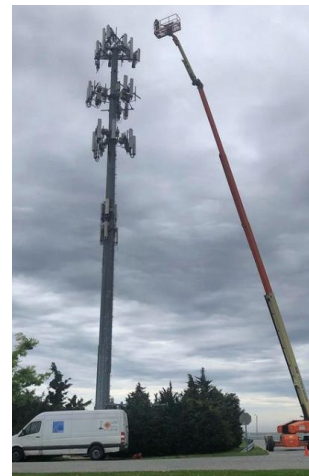
Figure 3-18, example of monopole tower
