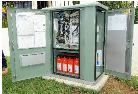
Figure 3-8, example of cross connection box
