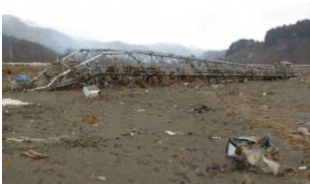
Figure 3-49, Cell site destroyed by the tsunami in Rikuzentakata
