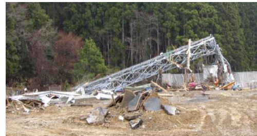
Figure 3-50, A collapsed tower of a base station located in the Karakuwa Peninsula.
