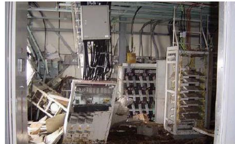
Figure 3-47, BSC components damage located in Iwate prefecture after Japan 2011 earthquake
