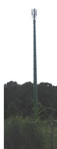
Figure 3-23, example of flanged monopole tower
