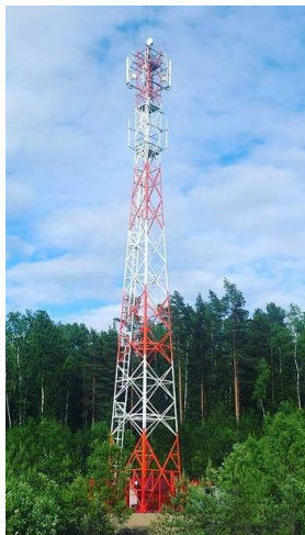
Figure 3-17, example of lattice tower
