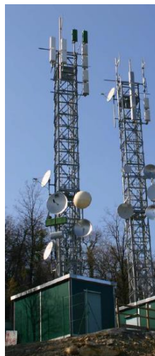
Figure 3-20, example of 4 sides lattice tower
