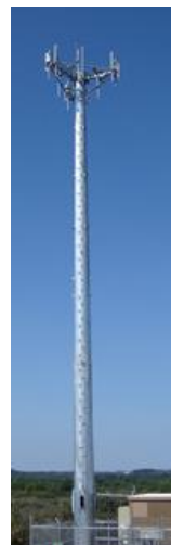
Figure 3-22, example of polygonal monopole tower
