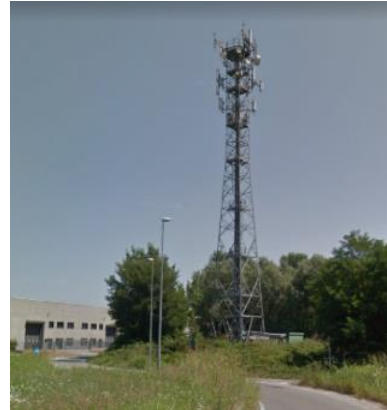
Figure 3-16, example of raw land BTS
