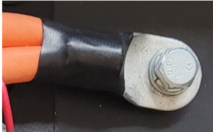
Figure 25 : HV cable ring termination
