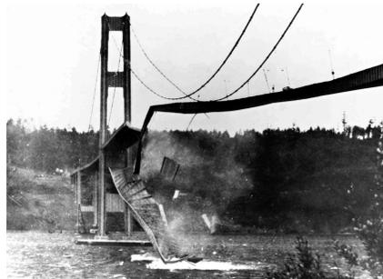
**Figure 2.3:** Tacoma Narrows bridge collapse in 1940 due to wind induced forced vibration
