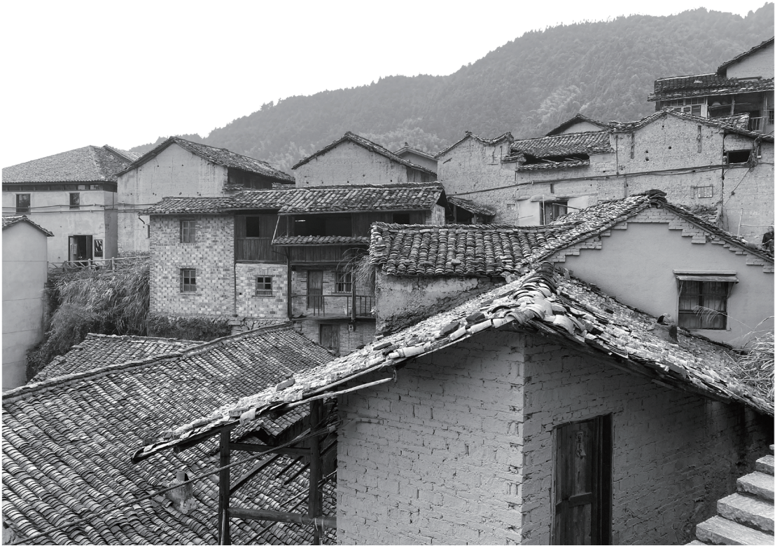
The mountain dwellings of Chenjiapu are surrounded by rammed earth on three sides, one side is close to the rubble retaining wall, and the internal roof truss is traditional wooden structure.
