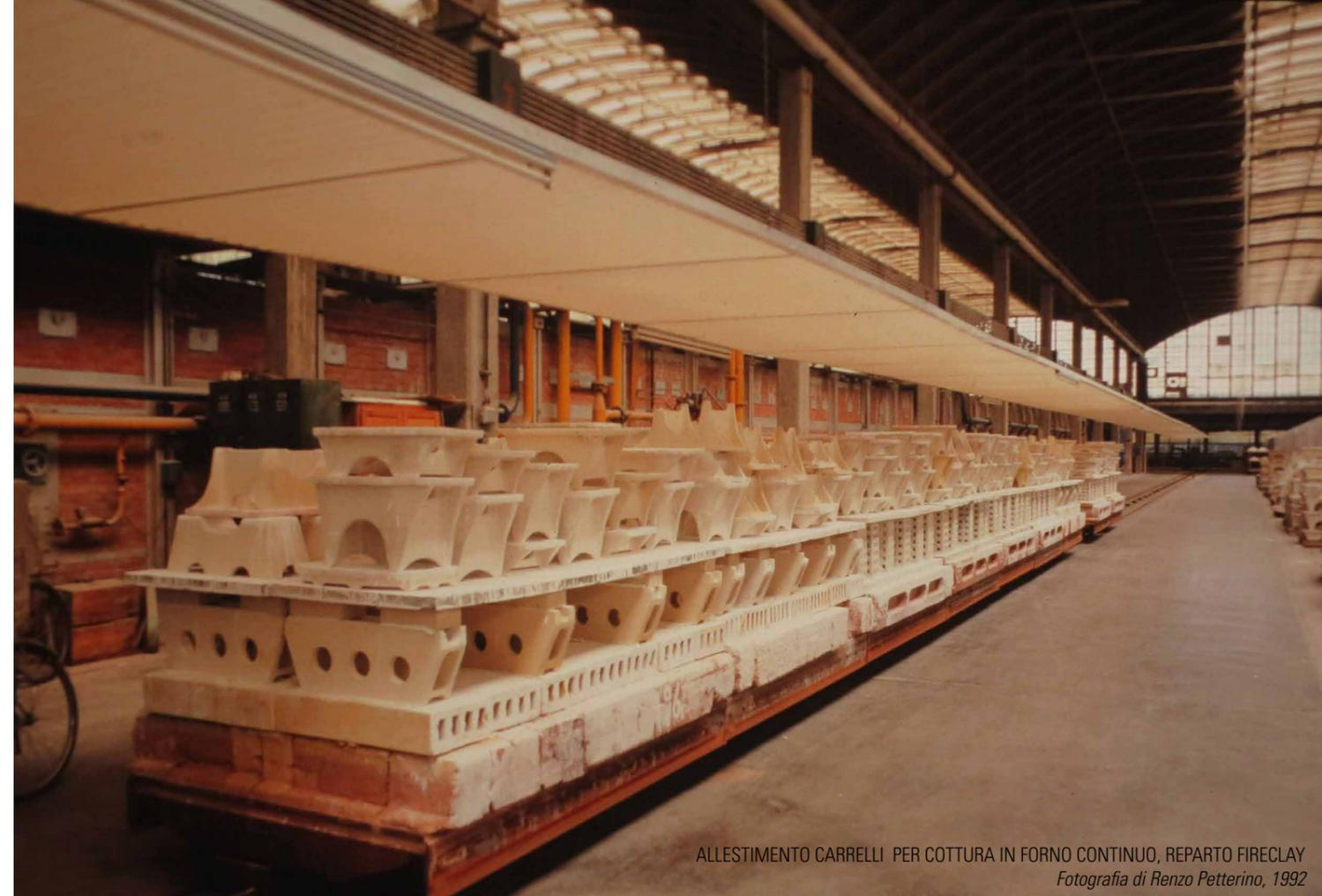
ALLESTIMENTO CARRELLI PER COTTURA IN FORNO CONTINUO, REPARTO FIRECLAY
