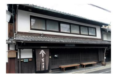
The façade of the house reflects the concept of a traditional machiya. The entrance has the large door with typical screens, allowing privacy. The thud stools are placed under the eaves. The roof is composed of sangawara tiles. The only difference is that the windows have been replaced with newer ones because they do not have the "insect cage".
