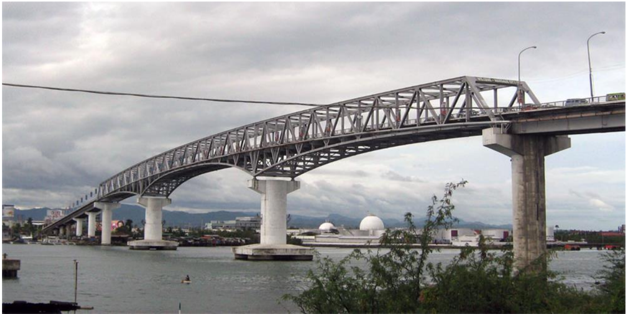
Figure 20: Sergio Osmeña bridge, truss structure
