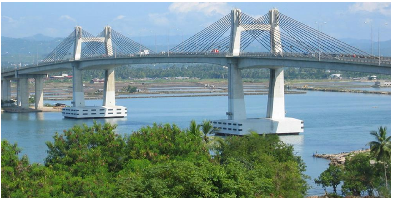
Figure 21: Marcelo Fernan bridge, extradosed cable-stayed structure
