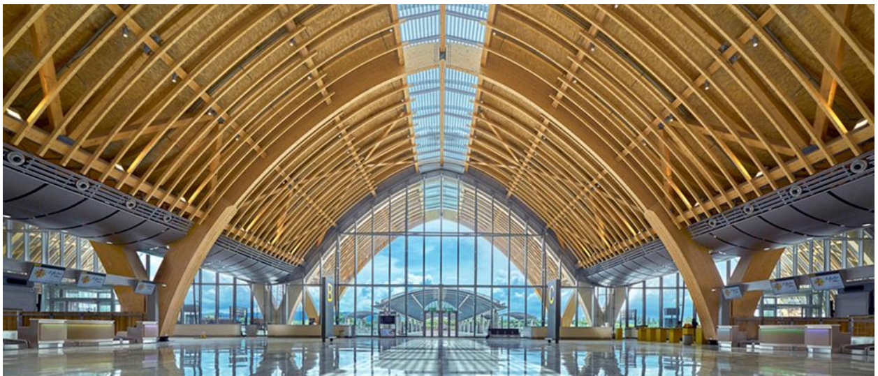
Figure 17: International Airport T2, timber arches structure
