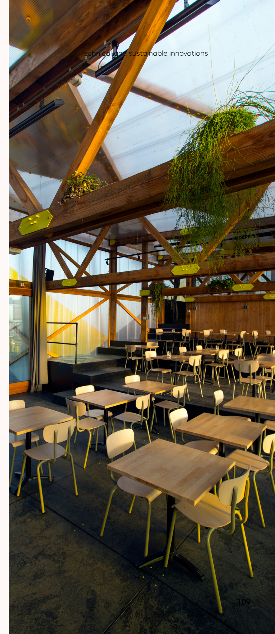
fig. 10 IRAUM Pavilion interior view: All the material inside is disassemblable, in line with the circular economy concept, © 2019, Deezen.com
