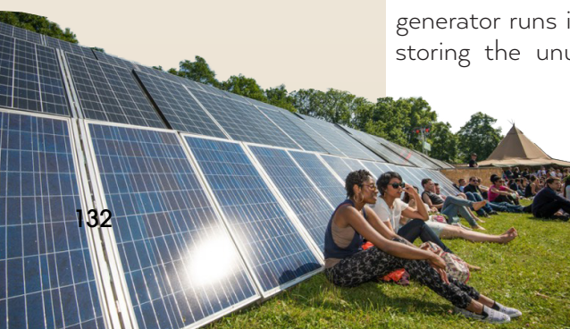
Fig. 6 The Solar panels installed by Firefly Clean Energy power supplier © 2014, Firefly Clean Energy organization
