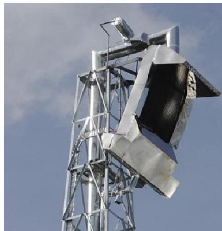
Figure 1.2 Jemalong solar thermal station: solar receiver on one tower.
