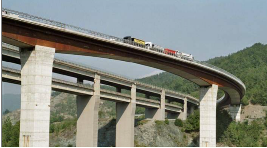
Figure 3.1: Overview of the bridge
