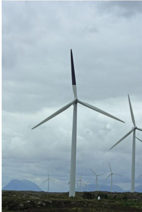
Figure A.21: Black paint on a wind turbine blade, image from [63]
