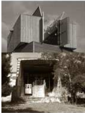
MONTE BIGNONE STATION
