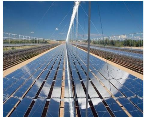
Fig. 6 Linear Fresnel Reflectors SolarPACES—Solar Power and Chemical Energy Systems
