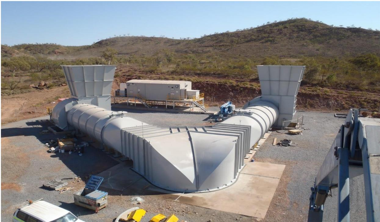
Figure 4.1: Mine primary centrifugal air fans (AIRENG Pty Ltd).
