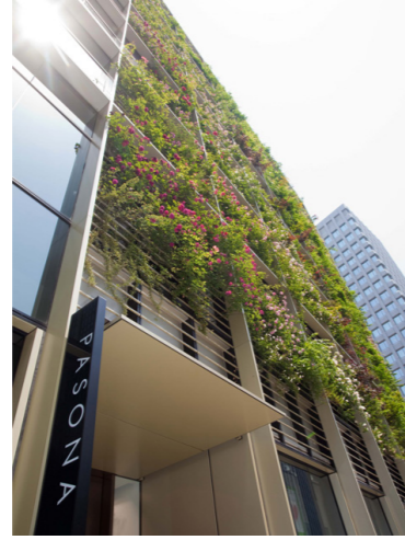
18. Pasona HQ Green facade
