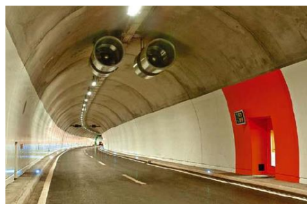
Figure 3.2: Couple of jet-fans for longitudinal ventilation system in tunnel.
