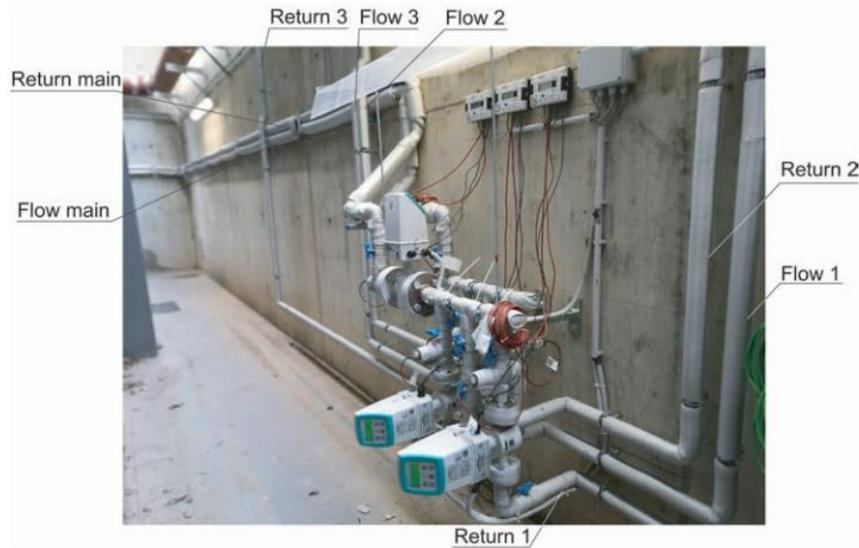
*Figure 4.6: Manifold connecting the pipes from/to the heat pumps with the heat exchanger modules (Baralis and Barla, 2019)*
