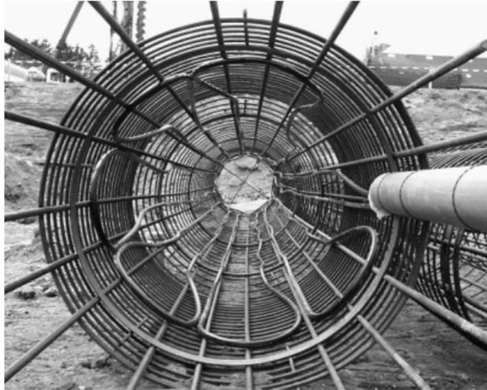
*Figure 3.2: Absorber pipes attached to the reinforcement cage (Brandl, 2006)*
