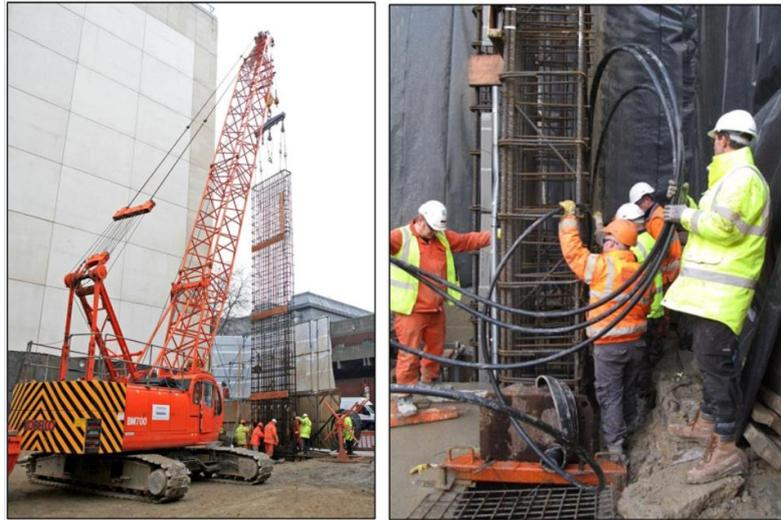
*Figure 3.12: Geothermal Loop and Reinforcement Cage Installation (Amis et al., 2011).*
