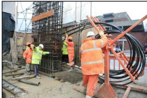
*Figure 3.11: Feeding Geothermal Loop onto Reinforcement Cage (Amis et al., 2011).*
