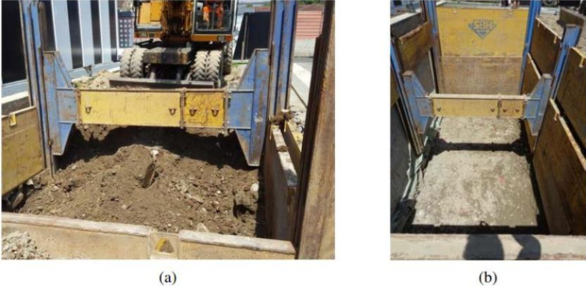
Figure 4.4: Trench shoring process: (a) early stage of excavation and (b) bottom of the excavation (Baralis and Barla, 2019)
