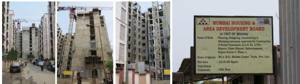
Figure 73- The process of construction of the experimental building
