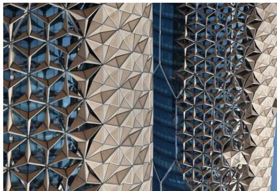
Fig. 41: Al Bahr towers shading system
