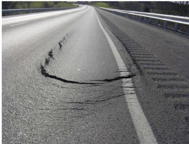
Figure 1.2: Slippage cracking on a surface of flexible pavement.
