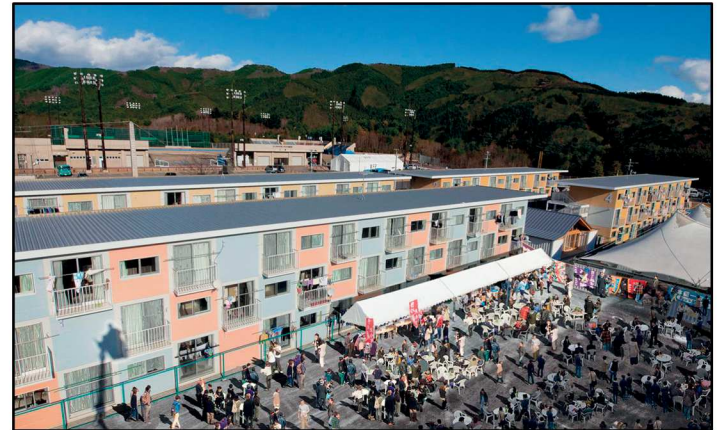
Fig.59 - Onagawa Container Temporary Housing -
