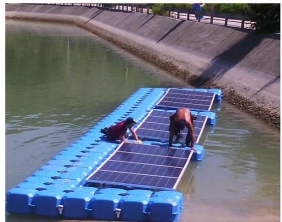
Figures 14-15: On the left NRG Island deployed letting the pre-assembled system slip on the shore, on the right a NRG Island system assembled on site, NRG Energia.
