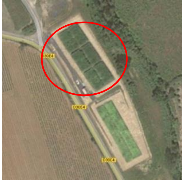
Figure 17 : The wastewater treatment plant seen from a satellite view
