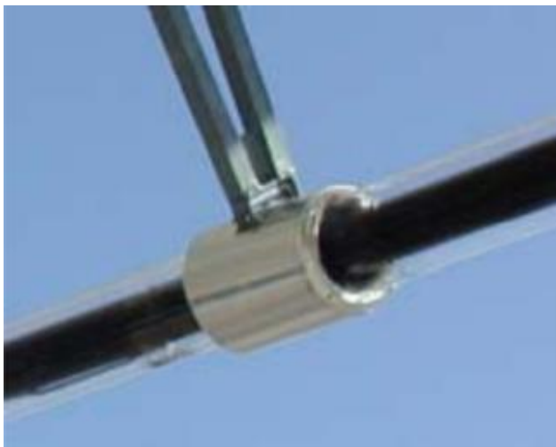
Figure 37 – Example of solar trough receiver support brackets [R. Forristall (2003)]
