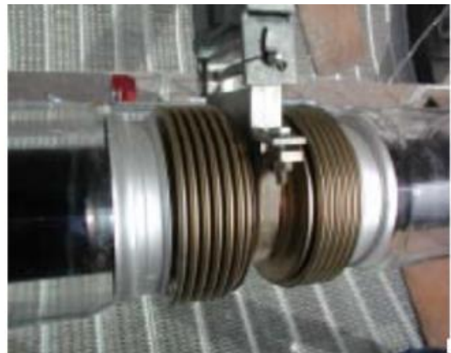
Figure 37 – Example of solar trough receiver support brackets [R. Forristall (2003)]
