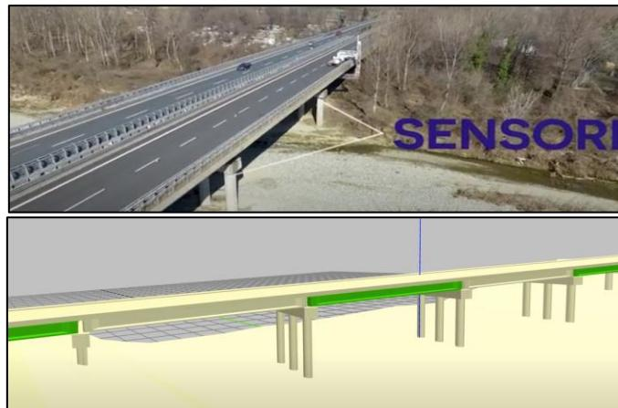
**Figure 18.** Location of the sensors previously positioned on the Stura Bridge and the model created. Source: ANAS S.p.A. and SYSDEV – Monitoraggio strutturale di ponti e viadotti.
