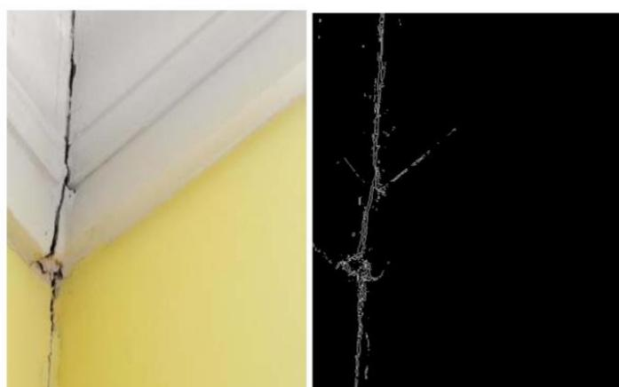
**Figure 2.** Example of automatized image processing for a crack wall. Source: Koshy et al., 2016. pp. 2
