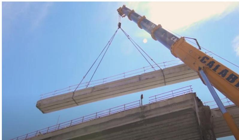
**Figure 12.** Largo Grosseto Overpass during its life service and during its demolition.
