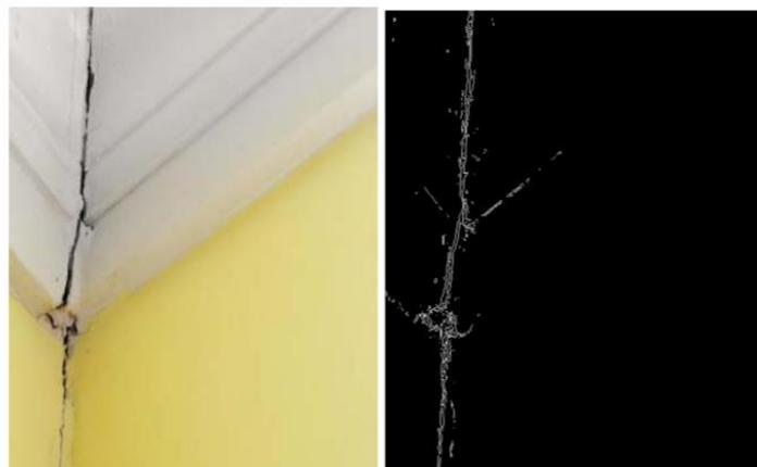
**Figure 2.** Example of automatized image processing for a crack wall. Source: Koshy et al., 2016. pp. 2
