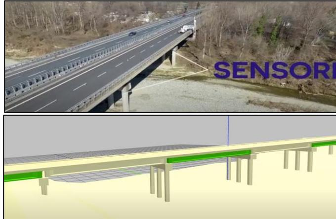
**Figure 18.** Location of the sensors previously position on the Stura Bridge and the model created. Source: ANAS S.p.A. and SYSDEV – Monitoraggio strutturale di ponti e viadotti.
