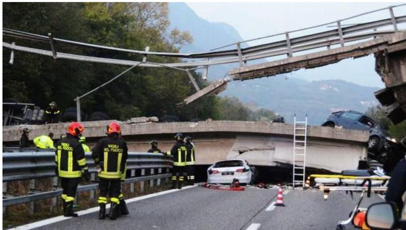
Figure 2.15: Annone overpass collapsed
