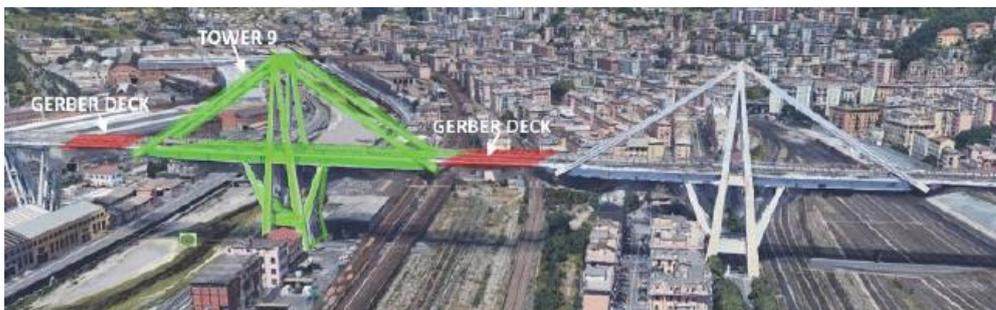
Figure 2.9: Polcevera viaduct before failure, highlight on Gerber beams and collapsed tower<sup>28</sup>
