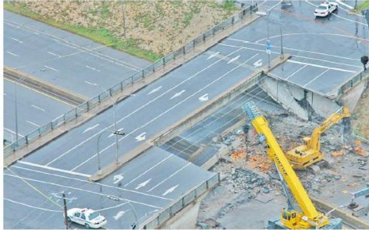
*Figure 2.12: The Concorde after collapse*
