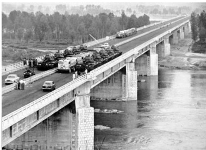
*Figure 1.1: Load test on the Po Bridge (Italy)*<sup>17</sup>
