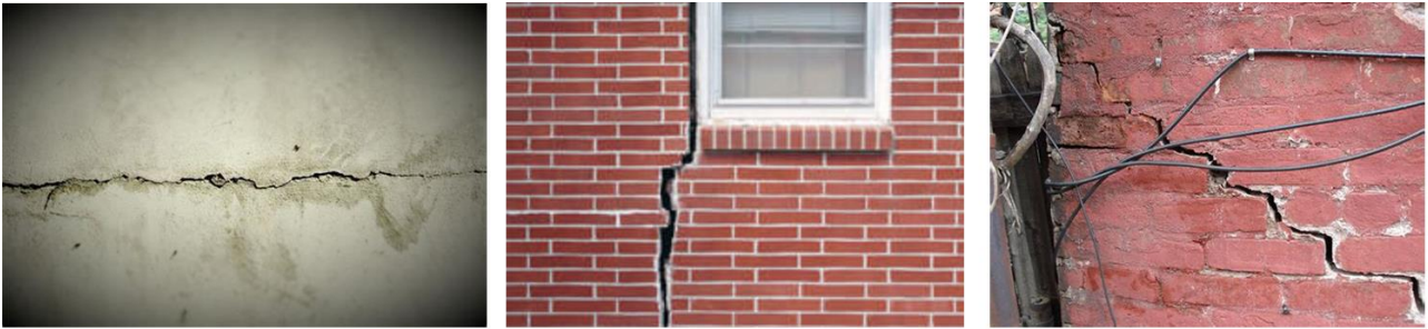
Figure 2.2 Different types of cracks depending on direction of propagation
