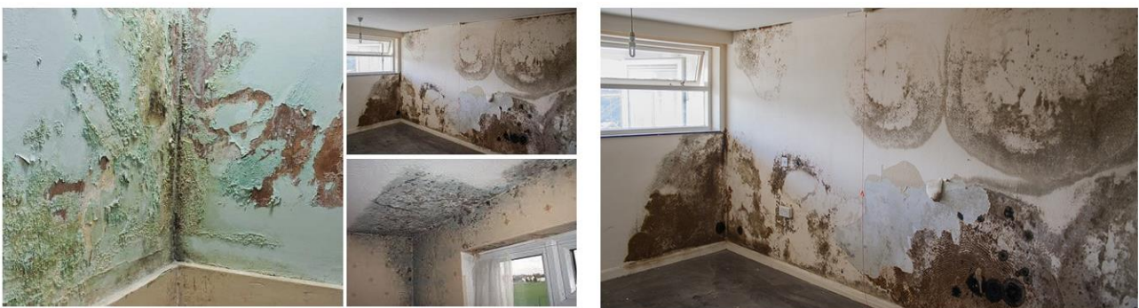
Figure 2.1 Damp-related defects
