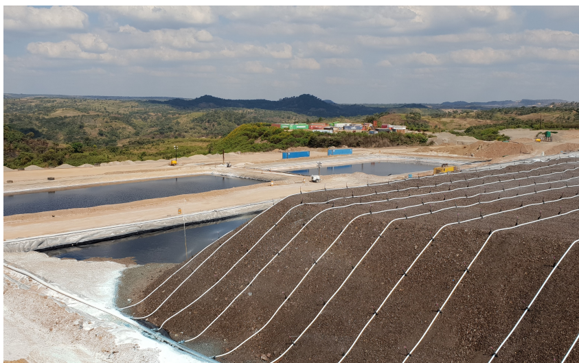
Figure 1.11. Heap leaching system, from Agua royal spring (2020) .
