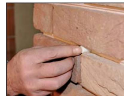
5. COPRIRE LE TESTE DELLE VITI CON I CILINDRI IN EPS PER EVITARE I PONTI TERMICI.
