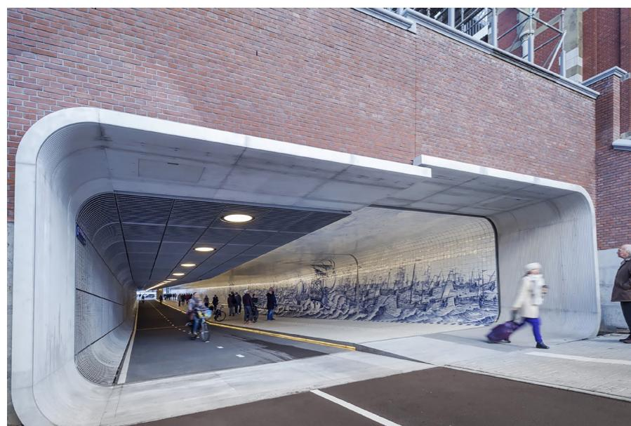
27. South side view, show how the pedestrian level is raised above the cycleway, allowing walkers to feel safe.
