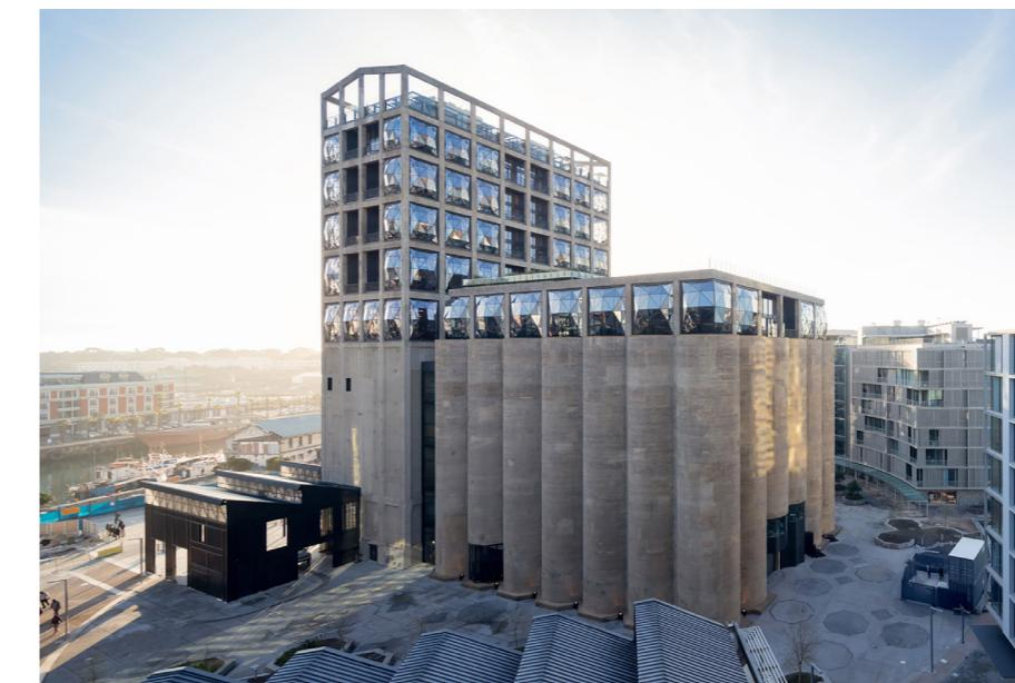
The interior spaces have been shaped inside the reinforced concrete supporting structure, reinforcements to the existing horizontal slabs (only 17 cm thick) have become necessary. These structural consolidations were followed by demolition works and cuts on the tubular structures in order to insert skylights and vertical connections, these works smoothed the entrance hall as a kind of cellular structure.<sup>48</sup>
