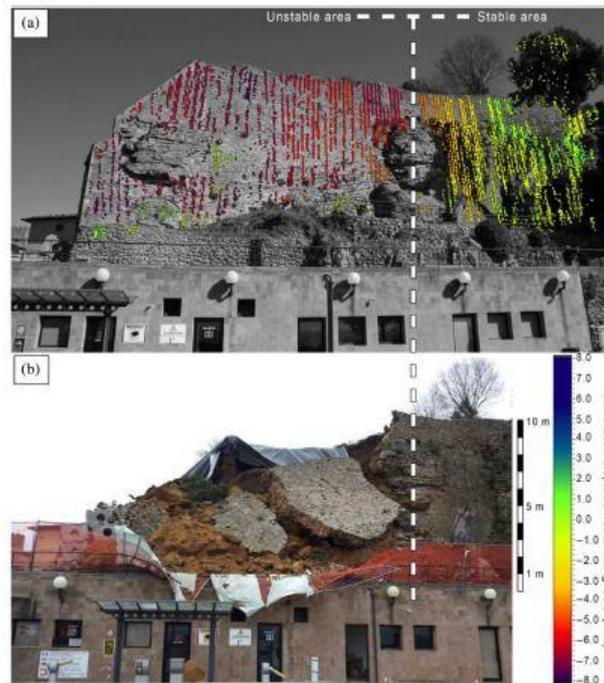
Figure 74: Prevision of walls collapse with LOS displacements, (Pratesi, et al., 2015).
